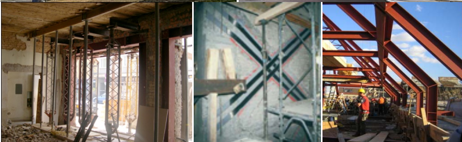
GENERALSANIERUNG WIEN 16 STRUCTURAL ENGINEERING RETROFIT ENGINEERING SEISMIC RETROFIT
