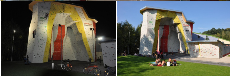
KLETTERPARK LINZ OUTDOOR CLIMBING WALL WANDFLÄCHE: 944 M 2
